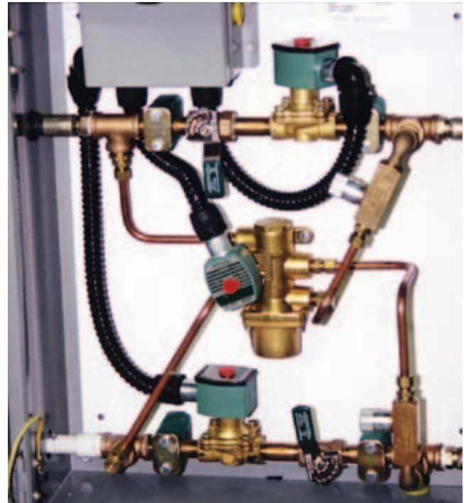
Pump check control system
