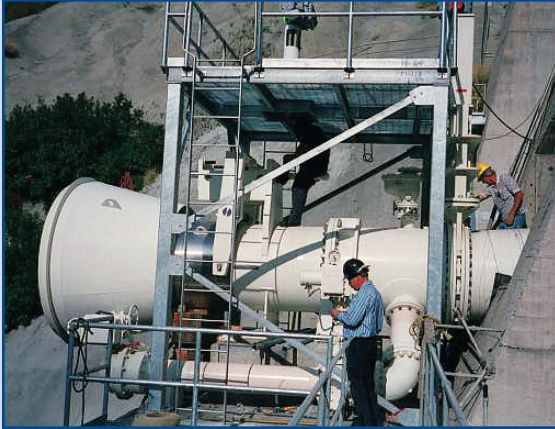
42" Fixed Cone Valve in a flood control application.
