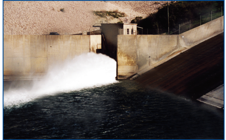
Free discharging fixed cone valve
