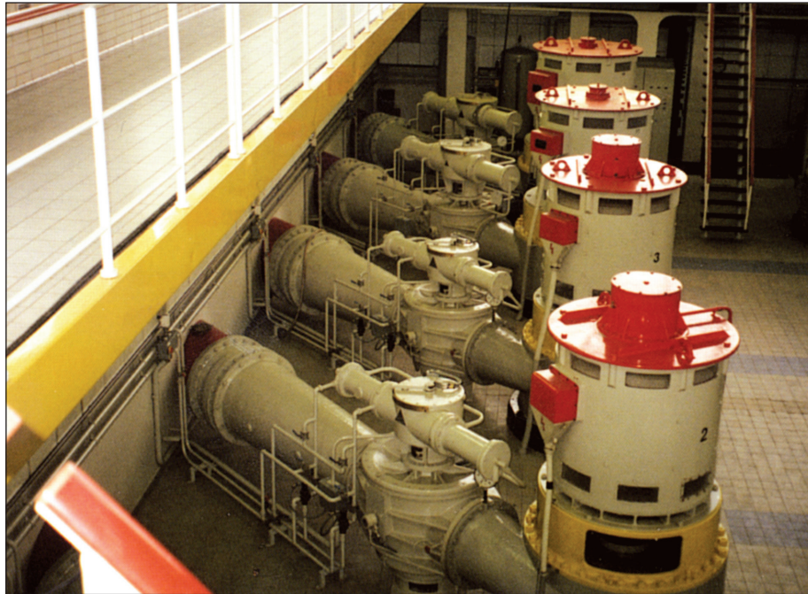
24" cone valves in operation since 1956.
