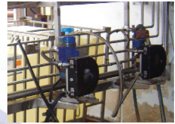
LSM-015 pumps for Acid and Caustic dosing in a CIP system
