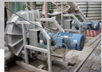
LSM-100 pumps installed in an African mining facility. Part of major order awarded due to the excellent features and superior hose life.
