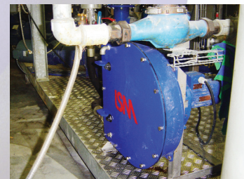
LSM Peristaltic Hose Pump with special coating. Beside Galvanized Steel and Stainless Steel, the pumps are available with special coatings for extremely harsh environments.
