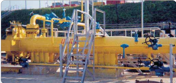
Client: SOFRESID SAIPEM France Location: Russia Pig Launcher "Beregovaya Compressor Station" Valves: DN 2" - 4" - 8" - ANSI 2500.
