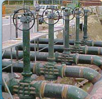
Client: SNAMPROGETTI Location: LOSTORF (CH) Valve: 20" Cl. 600 Venturi with Stem Extension.
