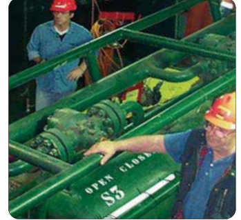
Client: SAIPEM - Italy LGTS - Green Stream Gas Pipeline Project Subsea Pig Launcher - Receiver Valves: DN 31/8" API 5000.
