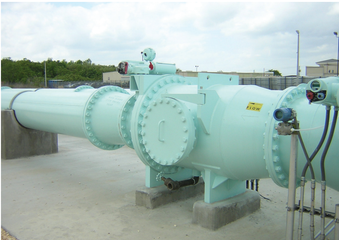
36" Model 711 Inline Sleeve Valve
